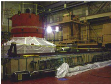
After removal of nuclear fuel, reactor vessel is shielded for decommissioning work
